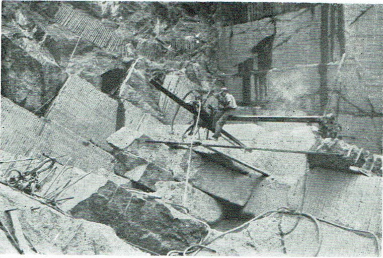
Fig. 2 A pneumatic drill mounted on an adjustable bar.
