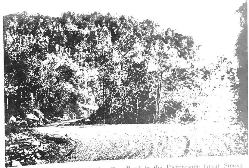
Fig. 6. A Portion of the Indian Gap Road in the Picturesque Great Smoky Mountains. Published through the courtesy of the Tennessee State Highway Department.
