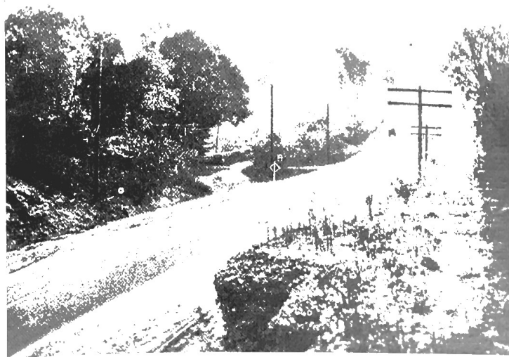
Fig. 4. An Excellent Asphalt-Surfaced Road on a Cement-Concrete Base, between Nashville and Lewisburg, Davidson County (State Route No. 11). Published through the courtesy of the Tennessee State Highway Department.
