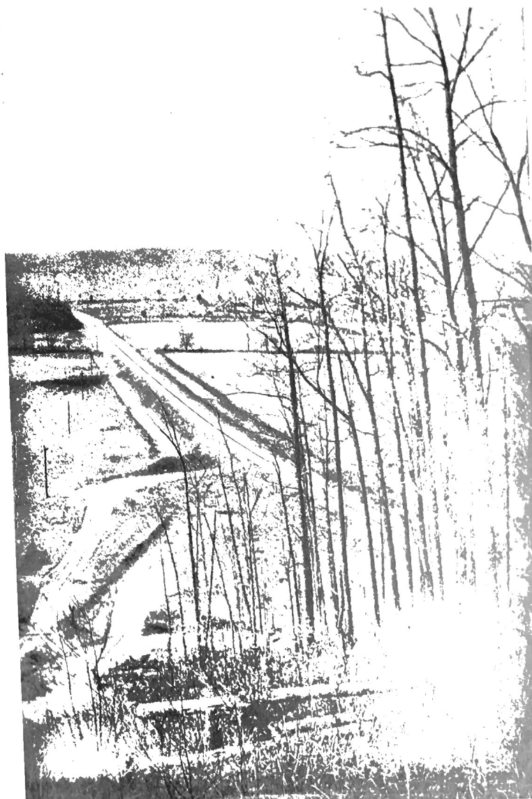
Fig. 2. A Beautiful Cement-Concrete Pavement between Waverly and Trotter's Landing Bridge, Humphrey County (U. S. Highway No. 70). Published through the courtesy of the Tennessee State Highway Department.
